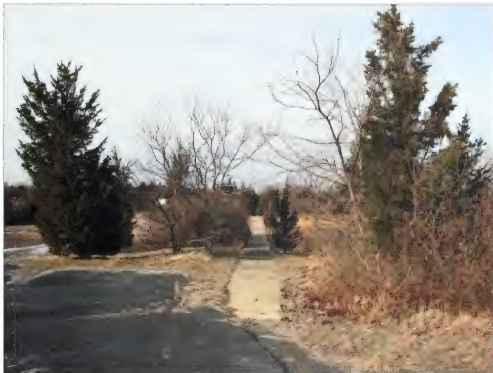
Figure 5.104. View looking north of sidewalk from Control Area #2 to the Ready Barracks, NIKE radar site. Asphalt, concrete, and gravel-surfaced circulation features should be cleared of woody vegetation six-feet off of all sides. Once woody vegetation, like the eastern red cedars seen in this photograph, has been removed, the six foot width can be easily maintained with a small tractor and brush hog mowing deck (Olmsted Center, January 2009).
